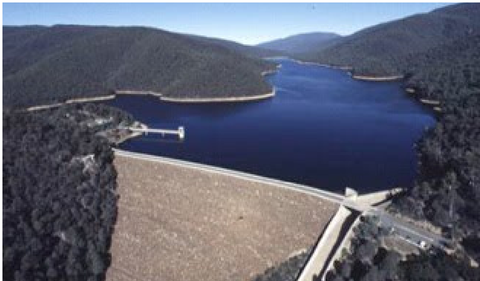
SIDE CHANNEL SPILLWAY DI BENDUNGAN HOPE, SCOTLAND
