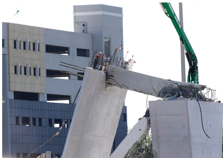
THE CRACKS IN THE CONCRETE AND STRESS MARKS IN THE METAL RODS
