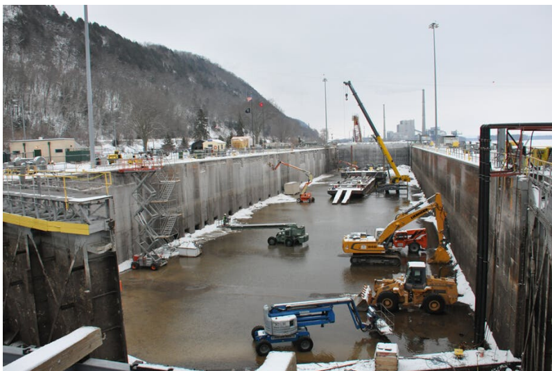
MAINTENANCE WORK ON LOCK AND DAM 8 ON THE MISSISSIPPI RIVER NEAR GENOA, WISCONSIN
